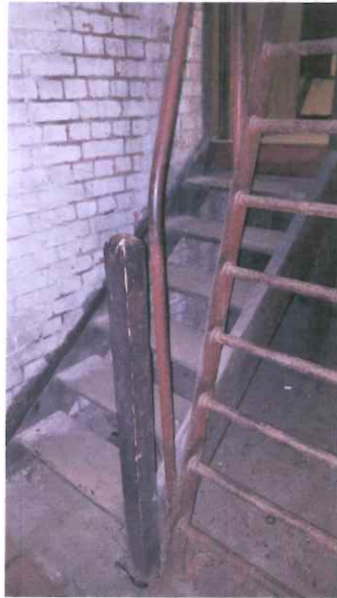
1.) Stairs to clock mechanism Ladders to floor above
