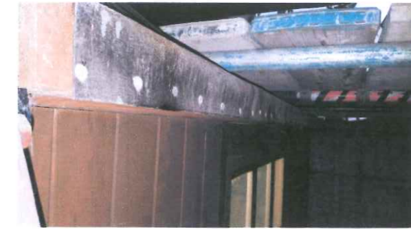
3.) Clock Mechanism roof with temporary scaffolding
